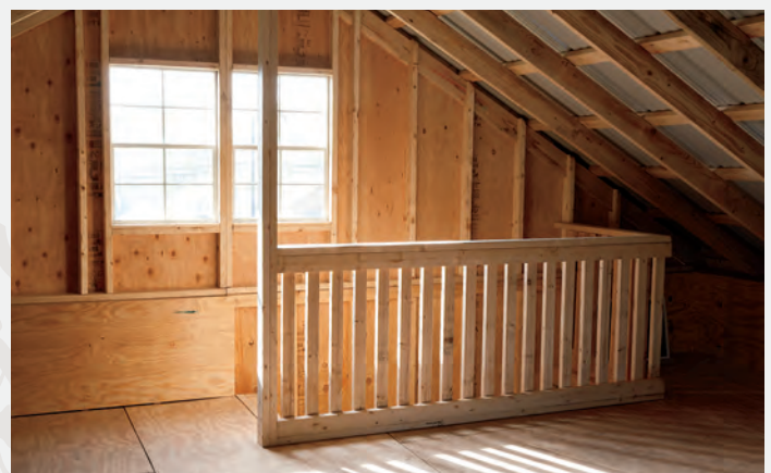
2 nd floor railings around stairwell
